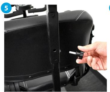
Install Long extension tube onto the top of the L shaped bar and fix into position with bolt and metal pin
